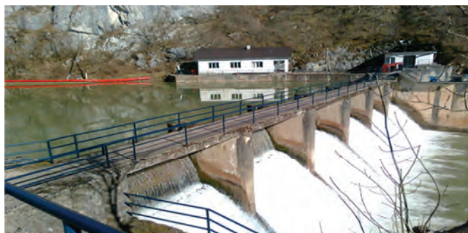
Fig. 3. SHPP Mesići dam [7]
