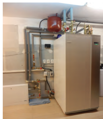
Fig. 2. Indoor Unit of HP system object A
