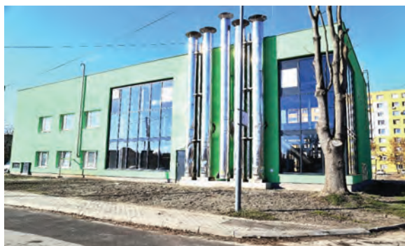
Fig. 7 – View to the reconstructed heat source – hot-water boiler house on natural gas.
